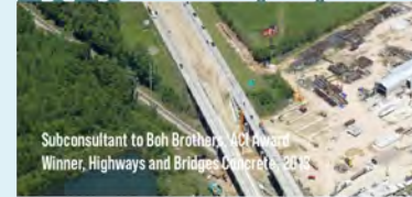
2013 I-10 Widening Design-Build
