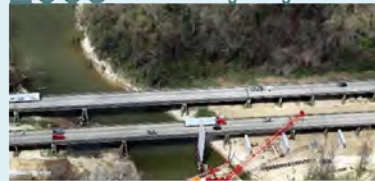
2009 I-12 Widening Design-Build
